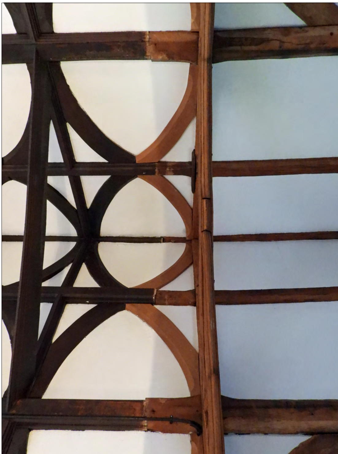
Repairs following the removal of the 1850 cross wall dividing the chapel from the accommodation to the west, showing as paler timber.
