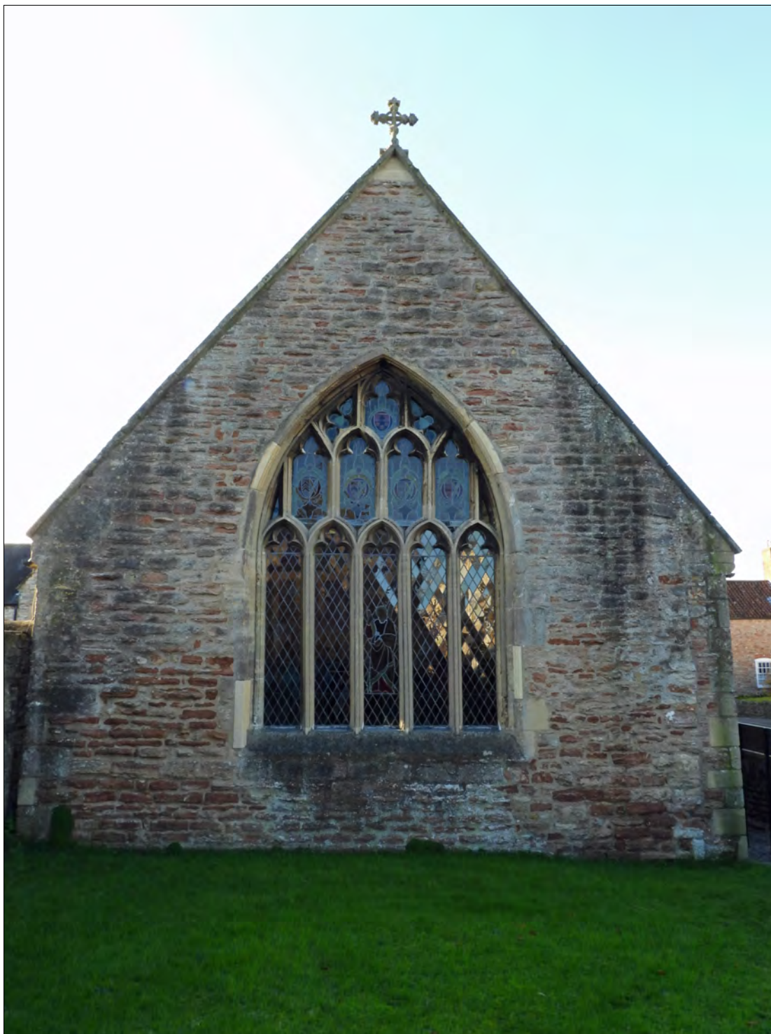
The East wall of the Chapel - the north-eastern quoin has been rebuilt - note the modern insertions around the window showing as paler blocks.
