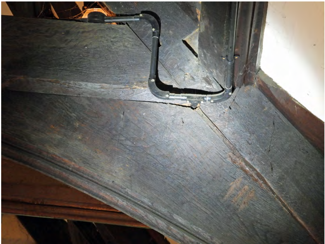
Carpenters' assembly marks, Truss 3 - north and south sides with differencing.
